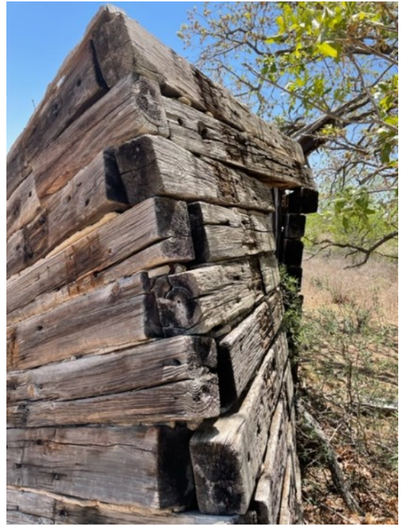
Log cabin” constructed from railroad ties probably built in 1960s. Site was one of three historic house sites recorded during May field trip to San Saba.
